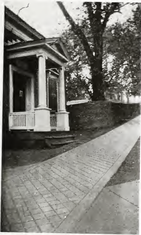
Porch Entering the "East Range," Where Poe Roomed; Serpentine Wall Beyond.
